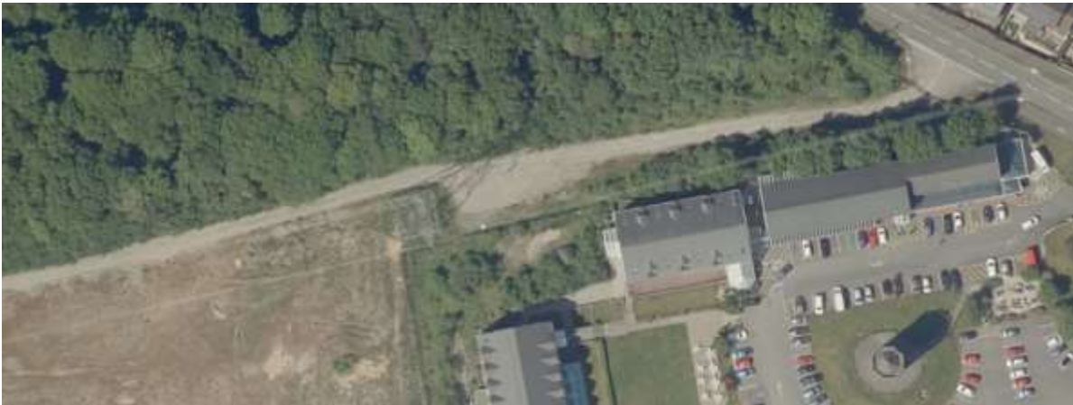
Figure 7: Existing Access to Site and Track
